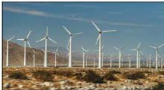
(g) Wind turbines
